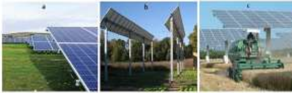
Figure 9: Installation heights of solar panels: a) Tradition way, b) and c) In the dual system
