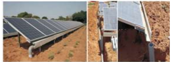
Figure 11: Rainwater harvesting system, source: [42]
