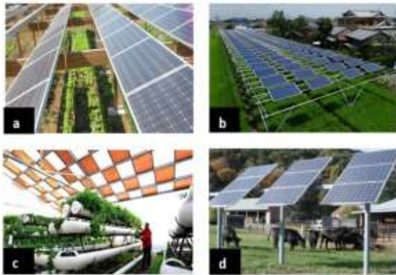
Figure 10: Possible field arrangements of PV panels a) Continuous rows, b) Staggered, c) Checker-board, d) Staggered
