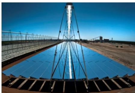
Figure 7. Schematic view of a typical LFR power system.
