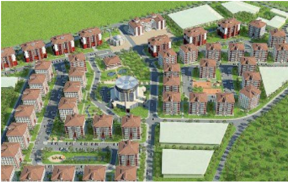
Figure 3: General view of the site.
